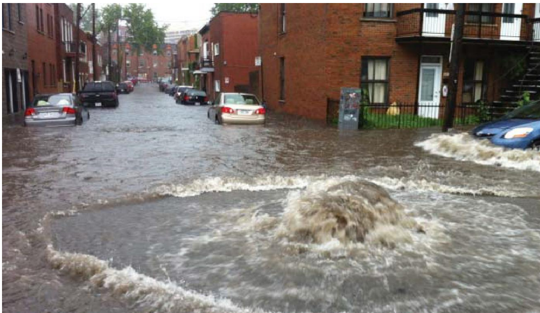
Figure 4. Sewer system overflowing after heavy rainfall in 2012. Source: Gilbert & Proulx, 2013
